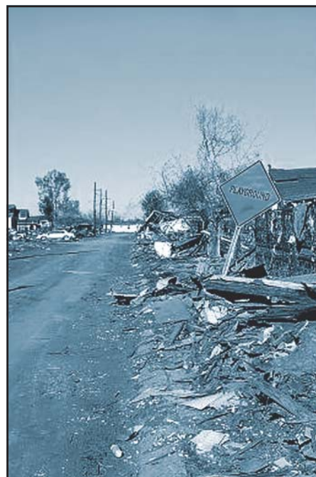
A street in the lower 9th ward.
